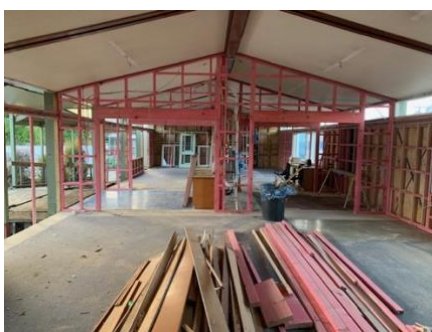
Block 5 from the inside with the new framework.
